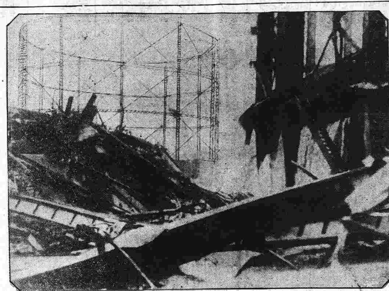
The scene of Pittsburgh's natural gas explosion disaster, photographed shortly after the blast, is pictured above. Havoc was spread throughout the lower north side industrial district of Pittsburgh when a tank containing 5,000,000 cubic feet of natural gas went off without warning. A score of men who were working on top of the tank were reported killed, with possibly a score more fatalities, many persons injured and homes, factories and other structures over a wide area wrecked.
